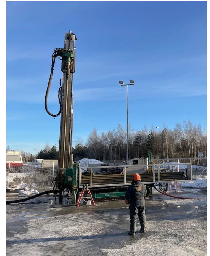
Drilling of 838-metre borehole near Tampere, Finland
